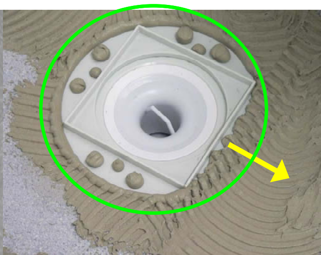
Free Floating Grate Retaining Ring (comes with 001.00034/5)
